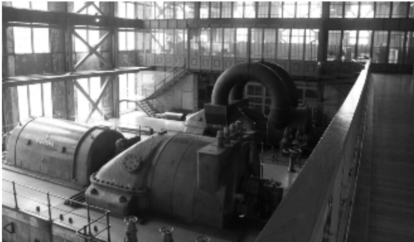
Figure 6: Control room behind the glass overlooking the machine hall
